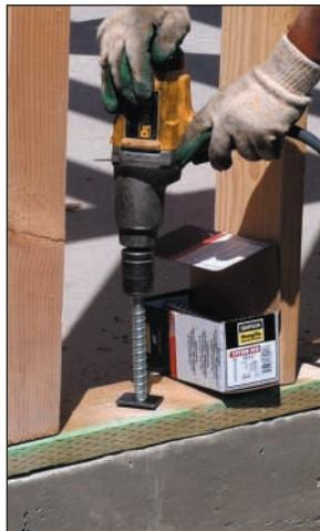
**TITEN HD® Heavy Duty Screw Anchor for Concrete and Masonry**
