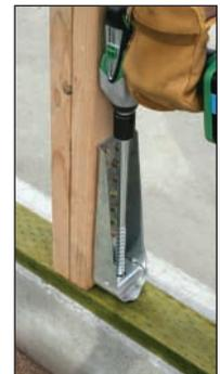
New longer 1/2" diameter Titen HD anchors achieve sufficient embedment depth to develop tension loads equal to many Simpson Strong-Tie holdowns that specify a 5/8" diameter anchor. Testing has been conducted to assure compatibility of these holdowns' anchor holes with the 1/2" Titen HD screw anchor.
