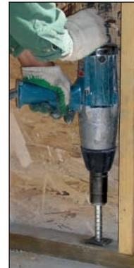
Suitable for use in place of code anchor bolts.
