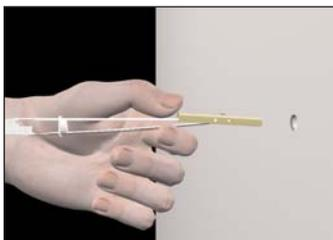
Drill appropriate size hole. Hold metal channel flat alongside plastic straps & slide channel through the hole. Minimum clearance behind wall: only 1 7/8".
