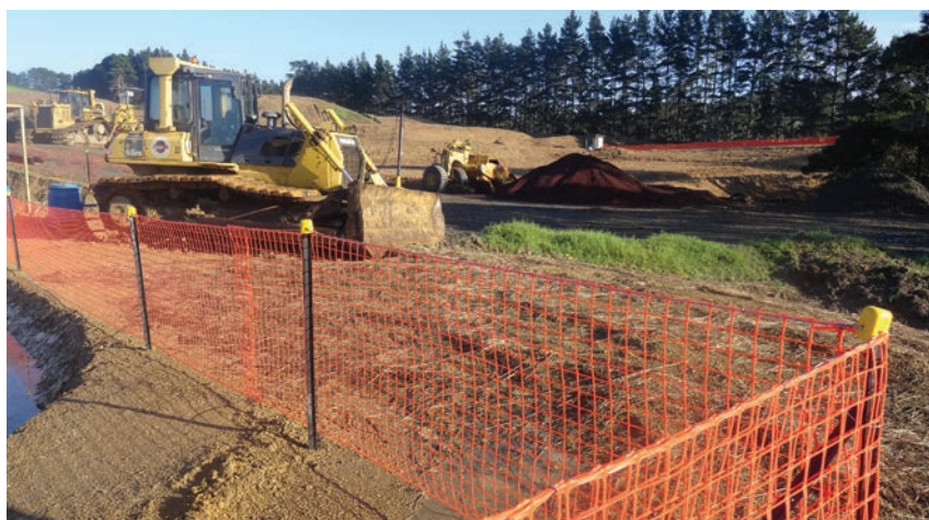
Fig. 25 Secure RainSmart system installation using barriers.
