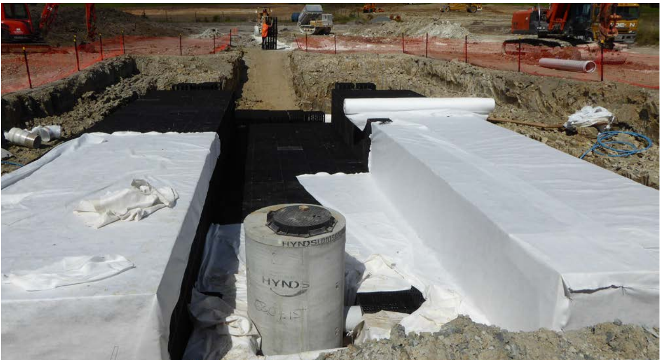
Fig. 18 Encapsulate RainSmart system with geotextile
