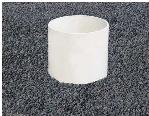
Fig. 17 Install port into RainSmart System
