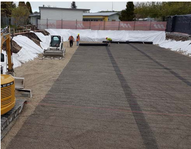
Fig. 24 Overlap geogrid 300mm or as required by plans.
