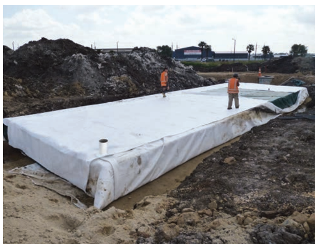
Fig. 16 Installed maintenance port
