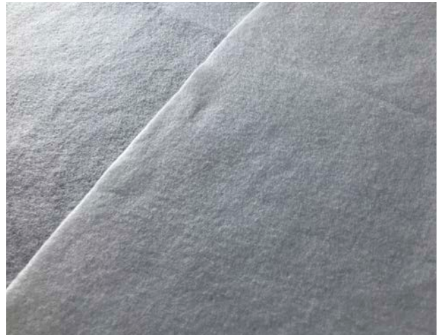
Fig. 7 Overlap geotextile by a minimum of 300mm
